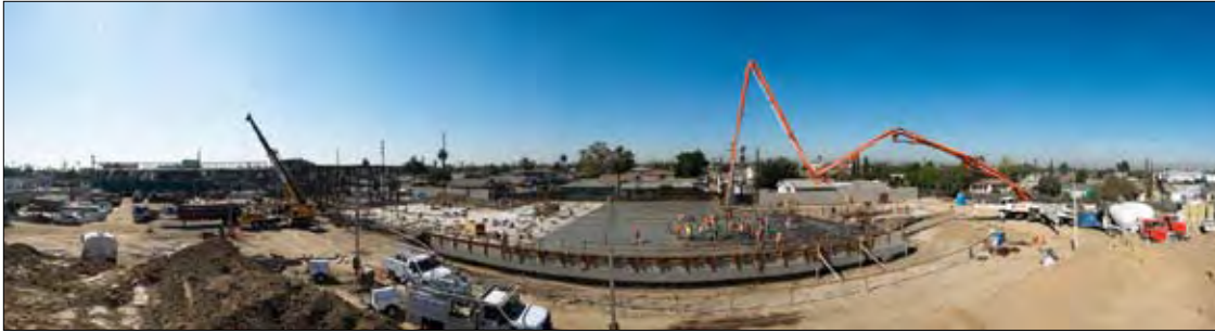
Panoramic view of progress on South Region ES #1
